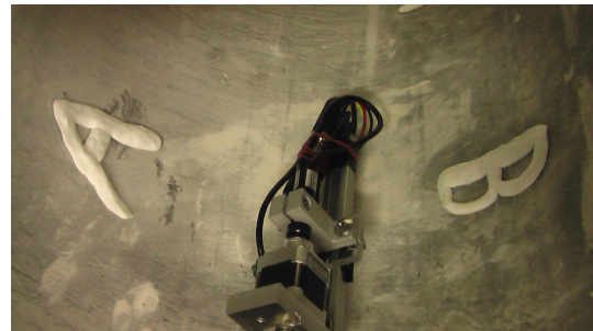
Fig. 17 Inside of the measured pipe
