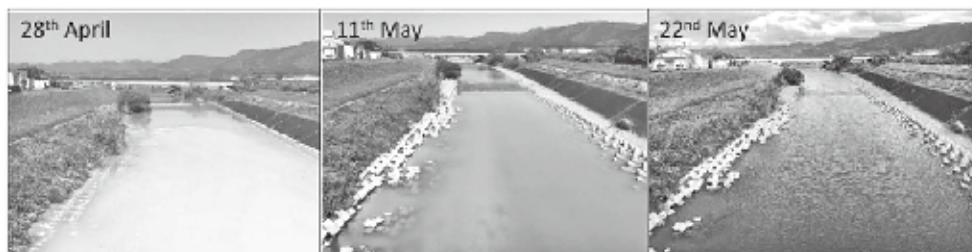
Fig.2 View of downstream at Nagae Bridge
