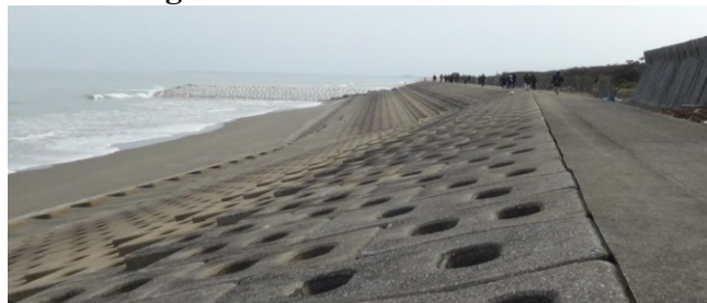
Figure 2.10 Gentle slope revetment
