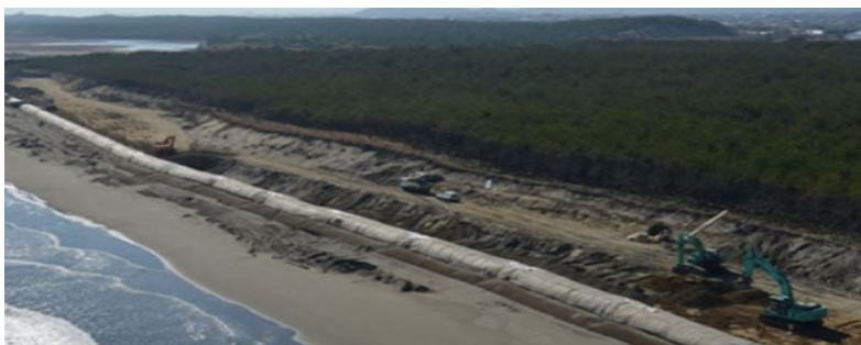
Figure 2.12 Sand-pack container and beach nourishment
