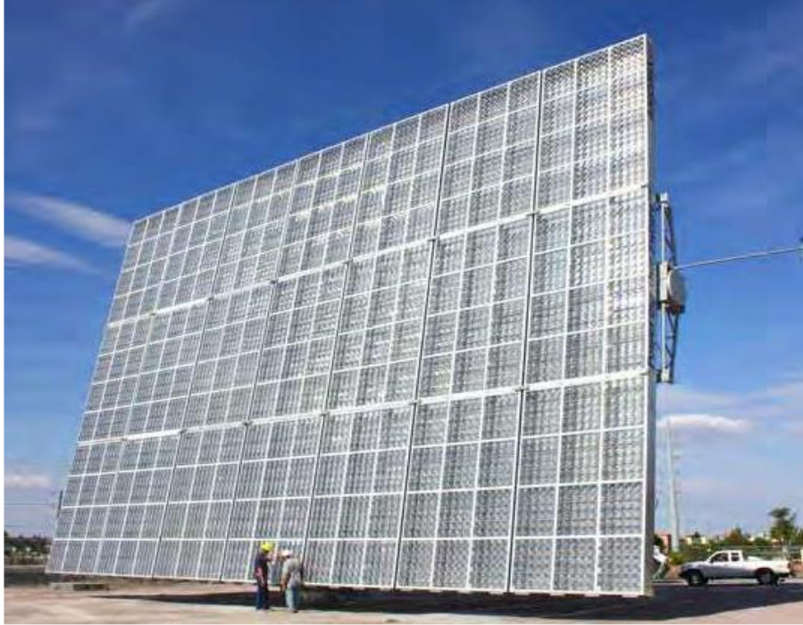
Fig. 1- 7: The Amonix 7700 60 kW AC system uses high-efficiency multijunction solar cells.
