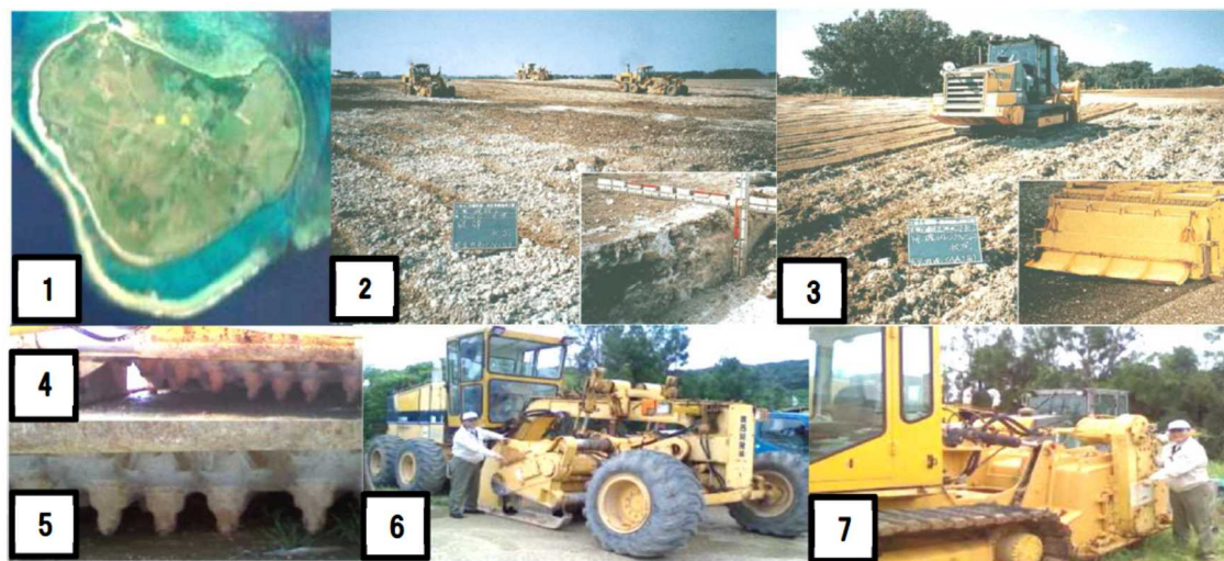
Photo 3 1: Kuro-shima from the sky, 2: Stabilizer method (40 cm depth) in 1992, 3: Stone crusher method (30 cm depth) in 1995, 4: Conical bits of Stabilizer, 5: Conical bits of Stone Crusher, 6: Stabilizer next to the author (1.75 m height) in 2013, 7: Stone Crusher in 2013
